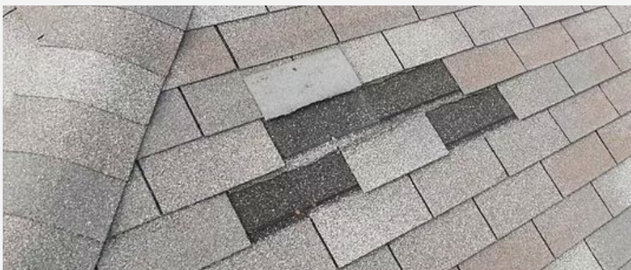
MISSING SHINGLES
